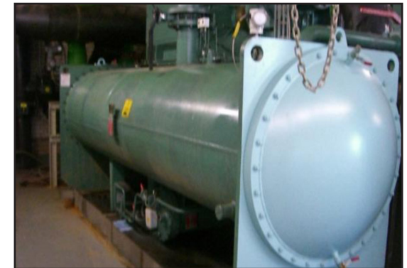
A regular maintenance check at 24 months showed no sign of corrosion or scale
